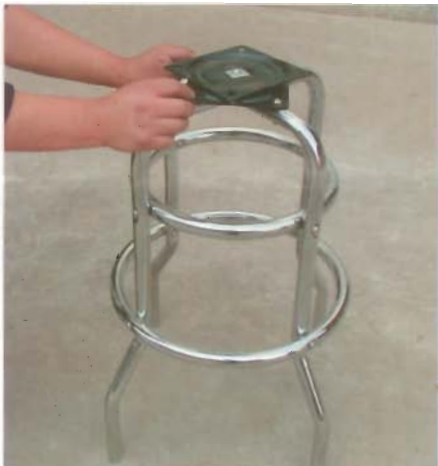
Step 4: Position the swivel plate on the top of the two barstool legs.
